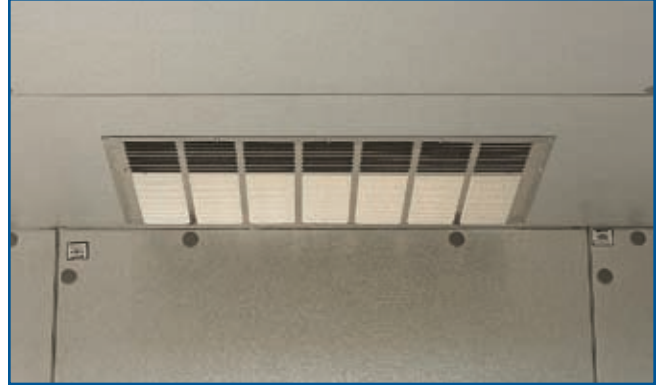
The PRS-2 evaporator grille mounts flush in a standard 4" thick panel allowing maximum storage space.
