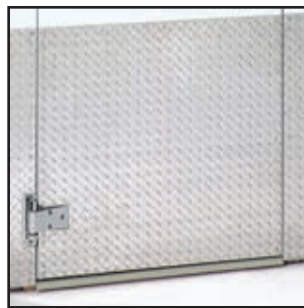
Kick plates protect doors and other panels from dents and scratches.
